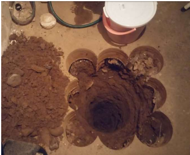
Figure 4.2. Excavation site used for CD injections at site Karjaa
