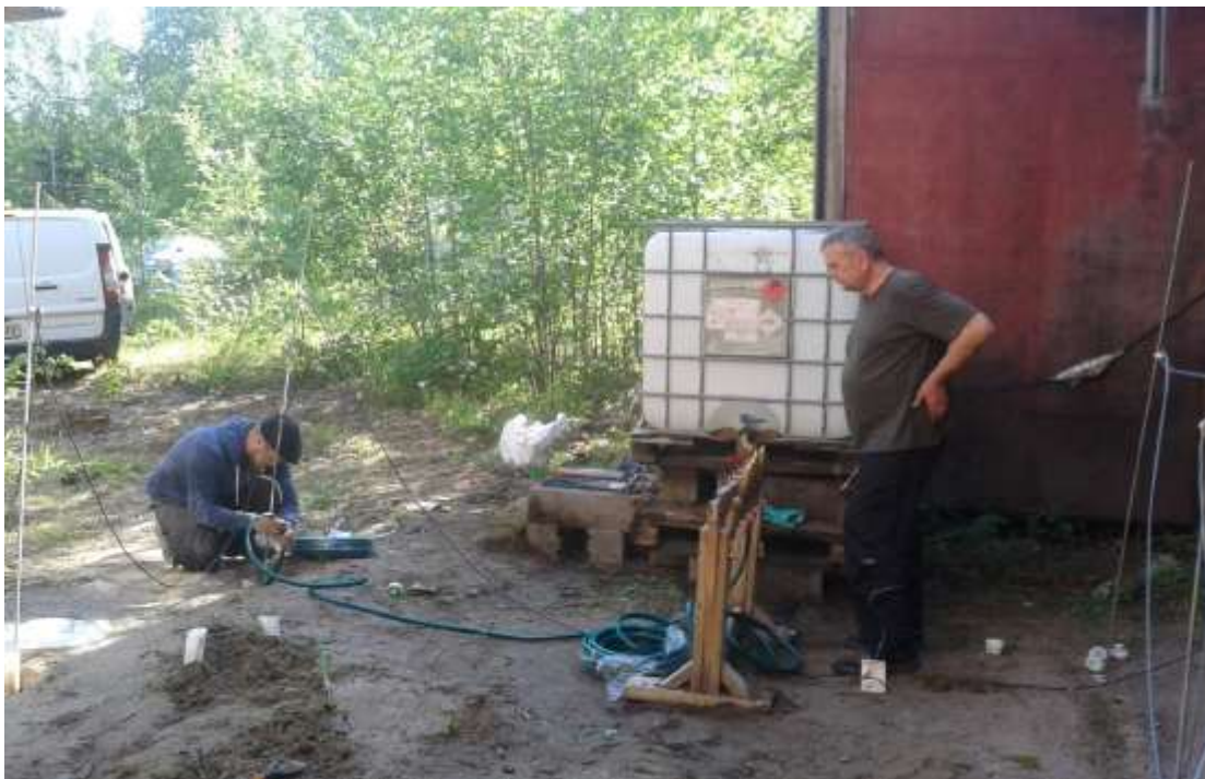
Figure 2.5. Installation of the water injection system.
