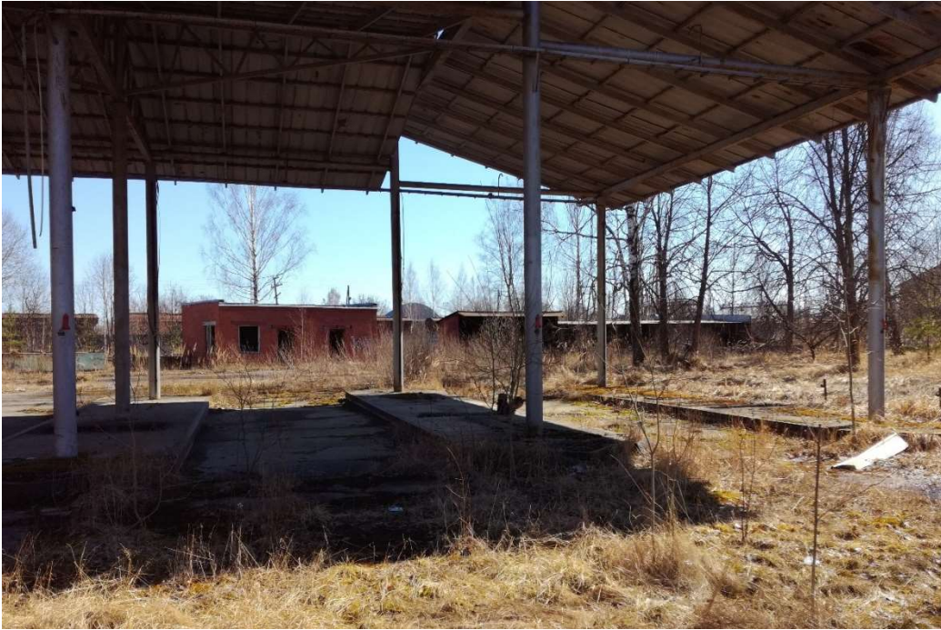
Figure 6.1. A former gas station and some abandoned buildings at the site Gaides iela.
