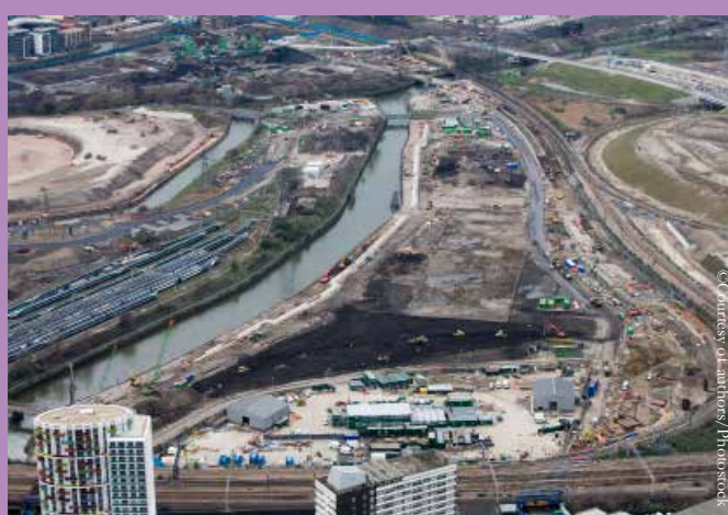
Aquatics site Enabling Works later.
