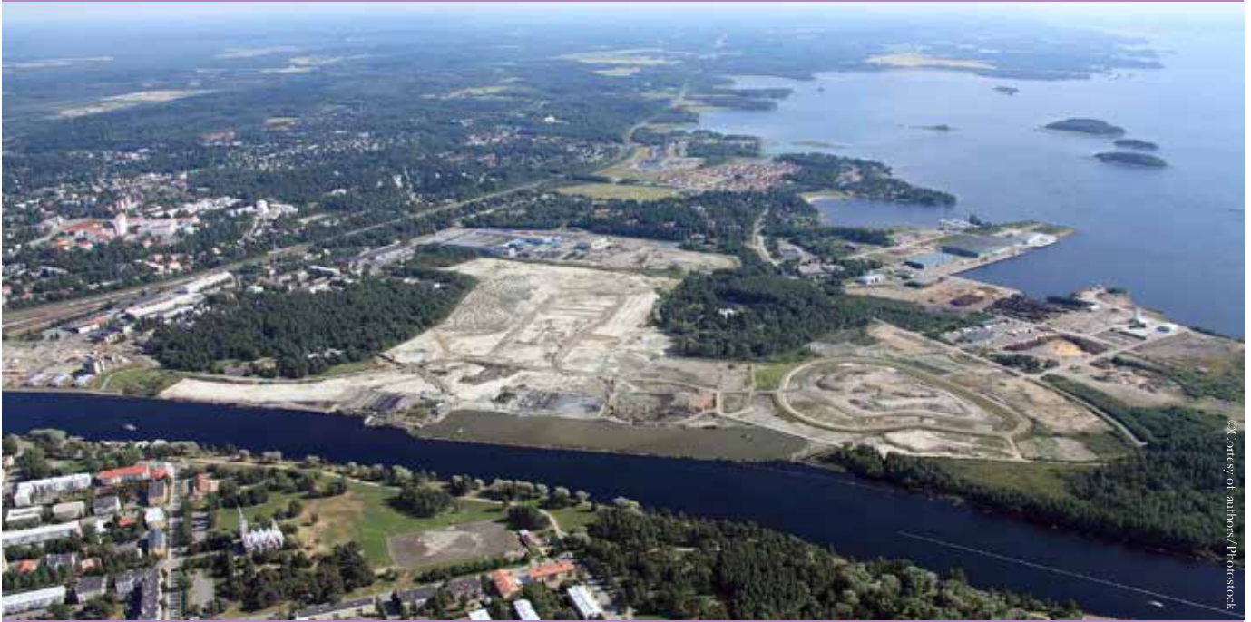
Aerial view of Penttilänranta area on the course of restoration works.
