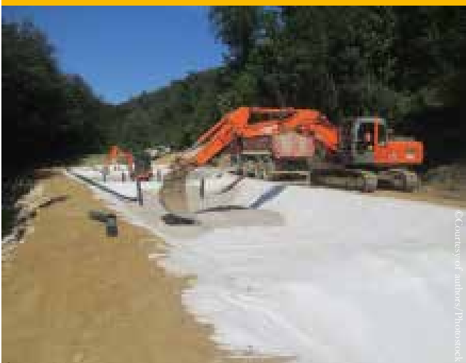
Preparation of limestone layer
