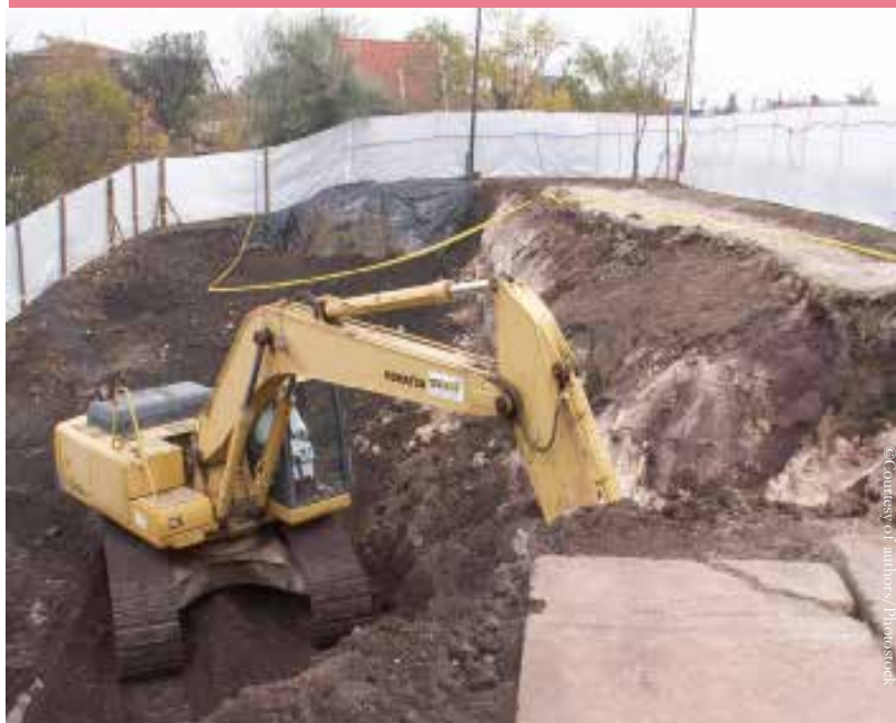
Excavation works on-site.
