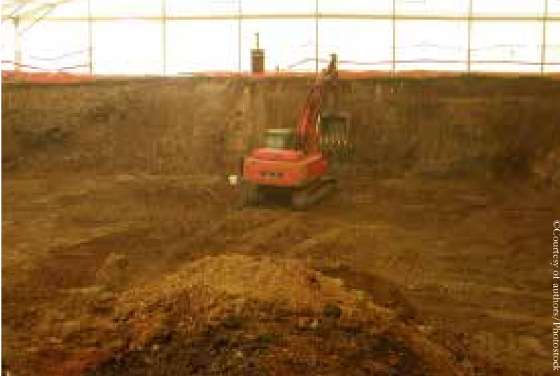
Excavation of most contaminated soil
