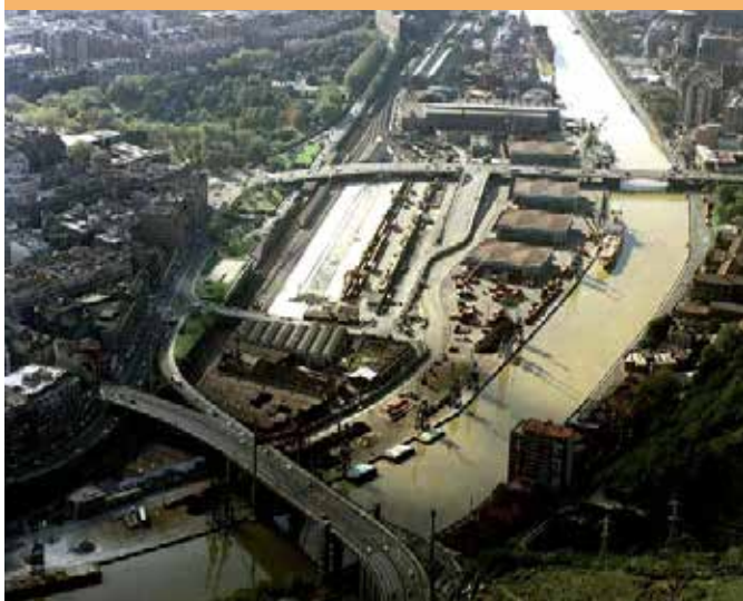
Area of intervention before remediation works, Bilbao river stuary.
