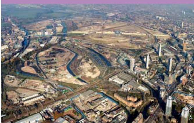
Enabling works aerial.
