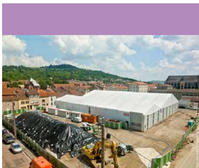
General overview of the site.
