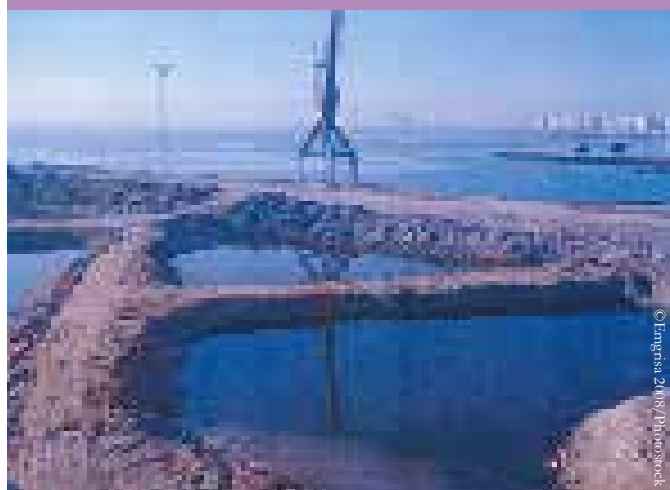
Stages of filling of lagoon 2 by the interposition of dykes
