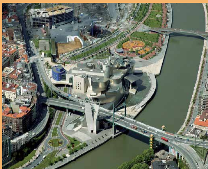
Area of intervention after remediation works, Bilbao river stuary.
