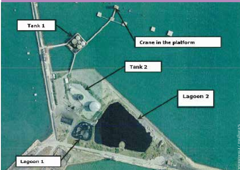
Aerial view of the plant before the remediation works.
