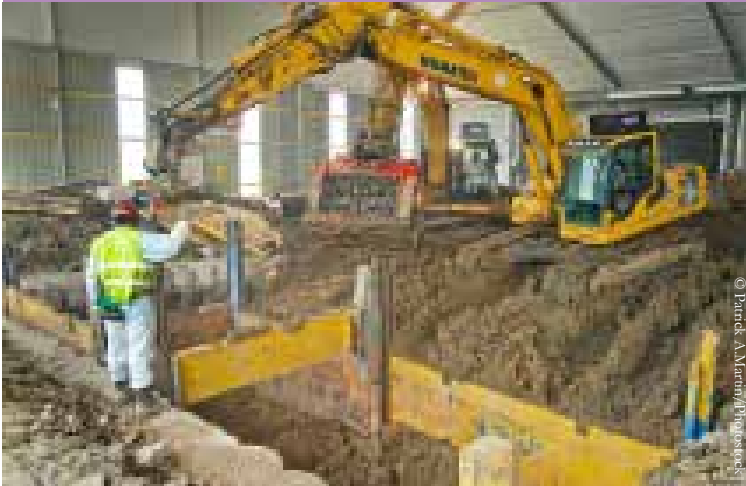
Excavation works under the confined tent.
