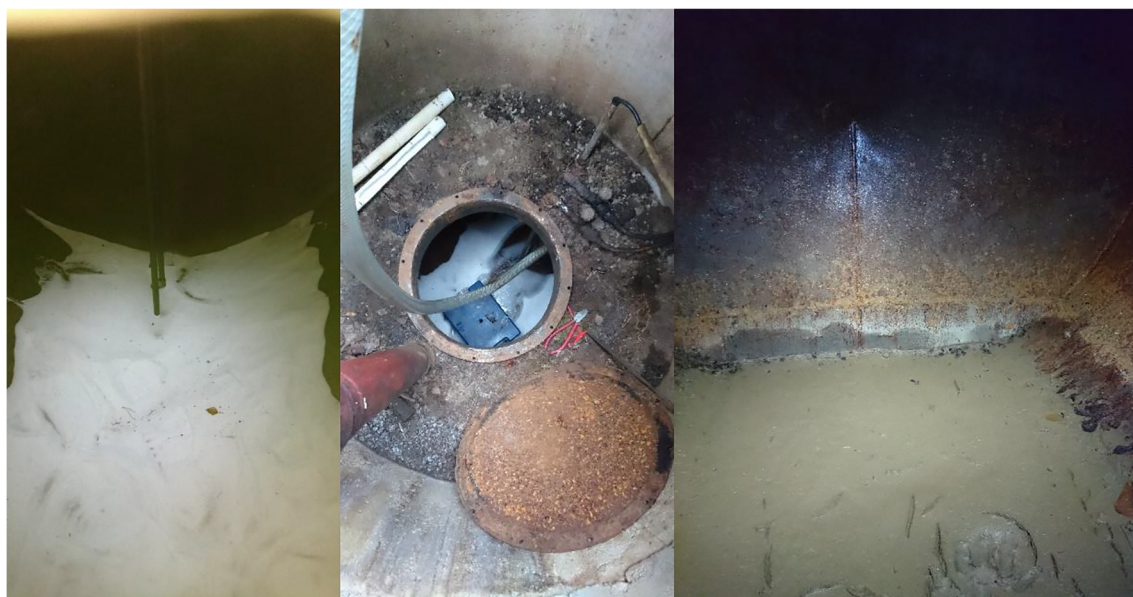
Fig. 4. Chemical treatment. Addition of citrate (a), injection of peroxide (b), resulting soil mobilization (c)
