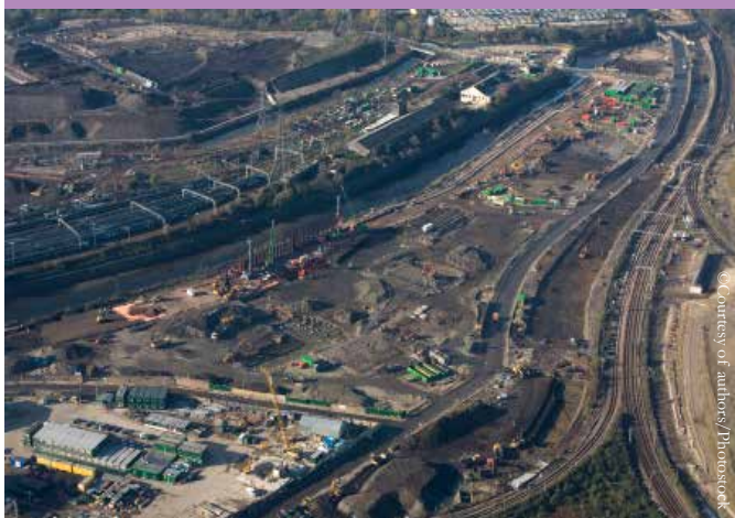
Aquatics site Enabling Works early.
