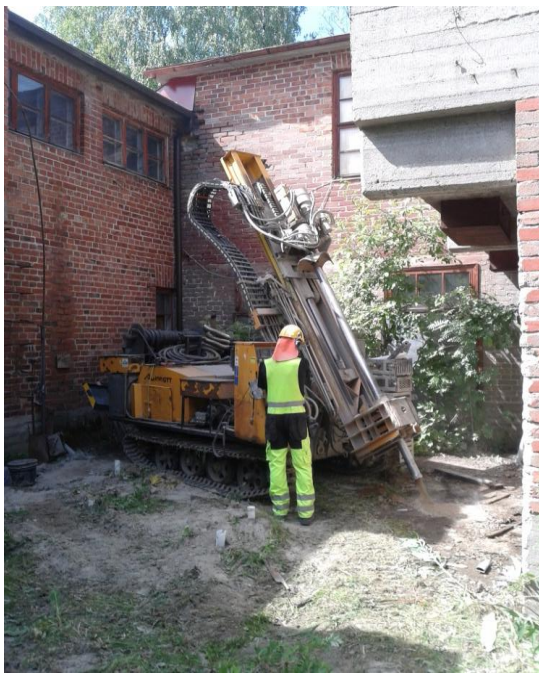
Fig. 4.1. Drilling/ installation of perforated tubes at site Nastola in June 2016
