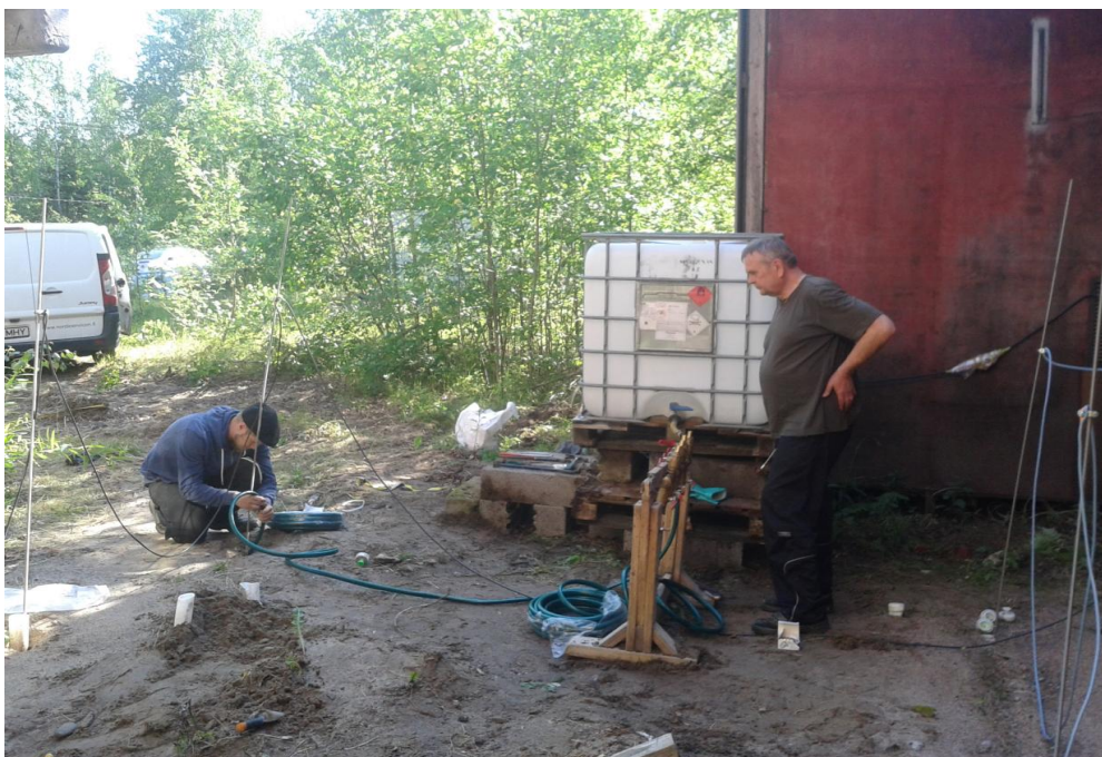
Fig. 4.3. Installation of the water injection system
