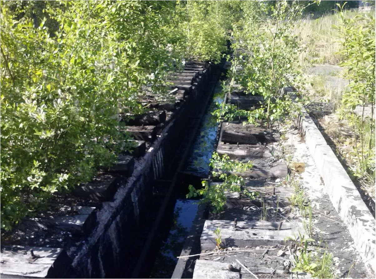
Figure 4. Residue of black fuel mixed with rain water near railroad branch for unloading of black fuel (May 2016)
