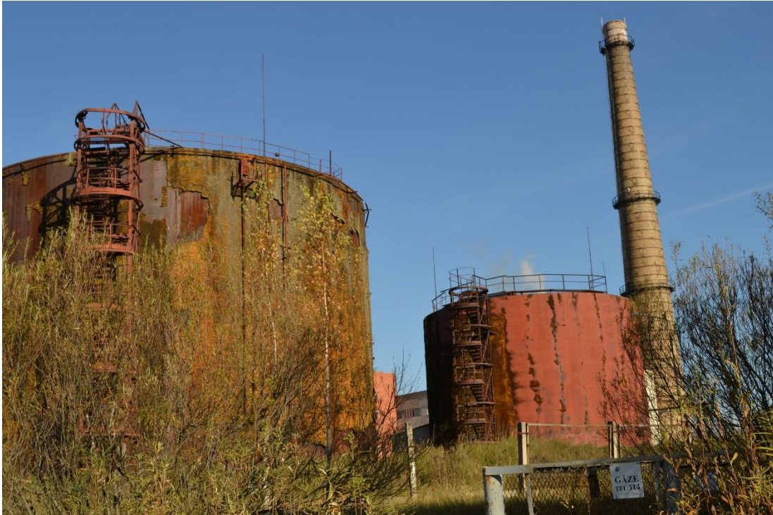
Figure 2. View on the former black fuel storage facility of Valmiera city heating company (photo from site visit in October, 2016)
