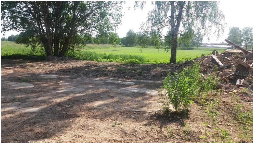
Figure 11. Building demolished, floor and debris left. Sight very similar to that what was observed in the site visit in October 2016. Crop field and main road can be seen in the background
