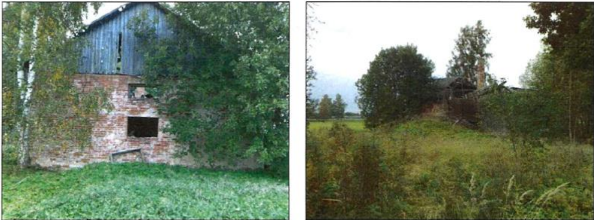
Figure 8. “Krustmaļi” agrochemical storage building (2012)
